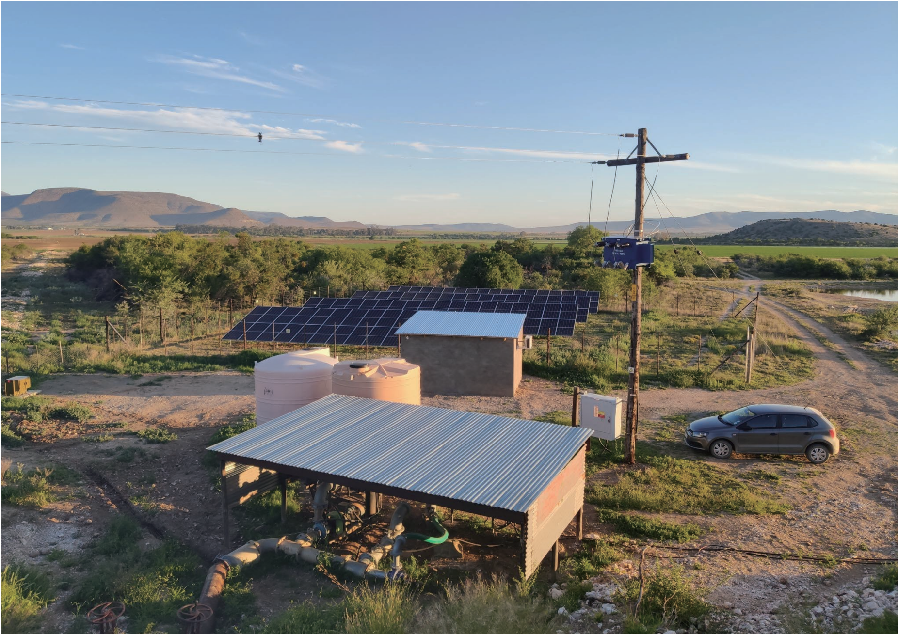
■ 50kW/200kWh+50kWp PV ■ 2023.10 ■ On/off-grid self-consumption
