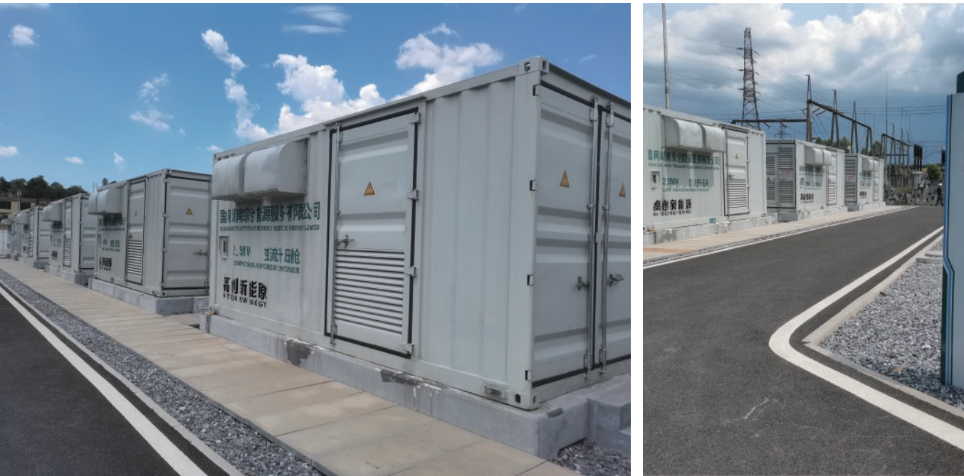
■ 100MW/200MWh ■ 2021.05 ■ Grid-side peak shaving and frequency modulation
