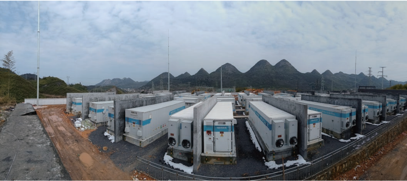
■ 100MW/200MWh ■ 2022.02 ■ Grid-side peak shaving and frequency modulation
