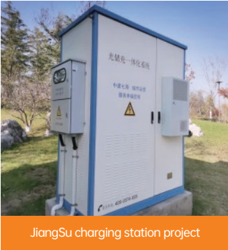
■ 300kW/650kWh ■ 2023.08 ■ Peak load shifting ■ JiangSu.china
