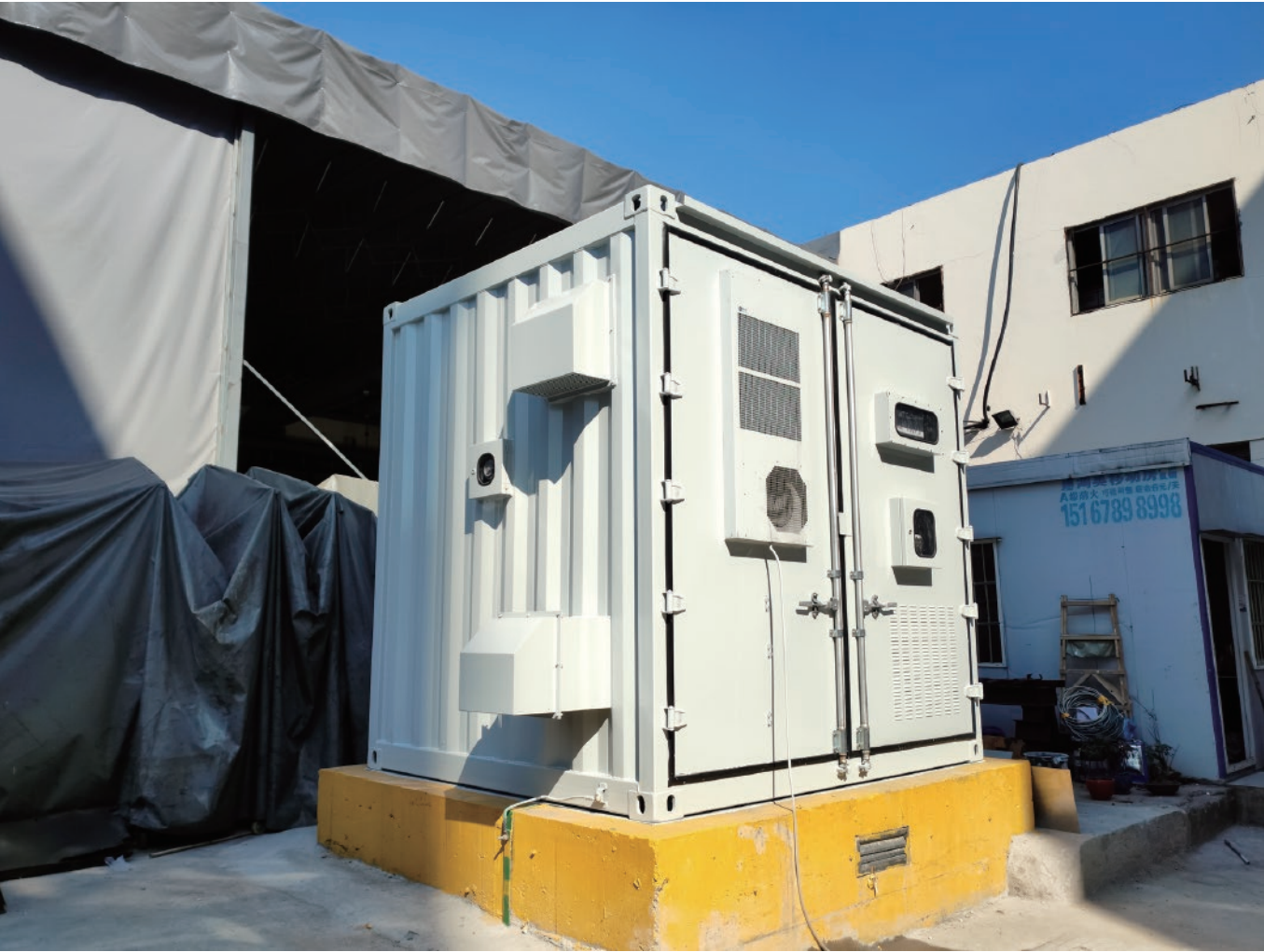
■ 300kW/650kWh ■ 2023.08 ■ Peak load shifting ■ JiangSu.china
